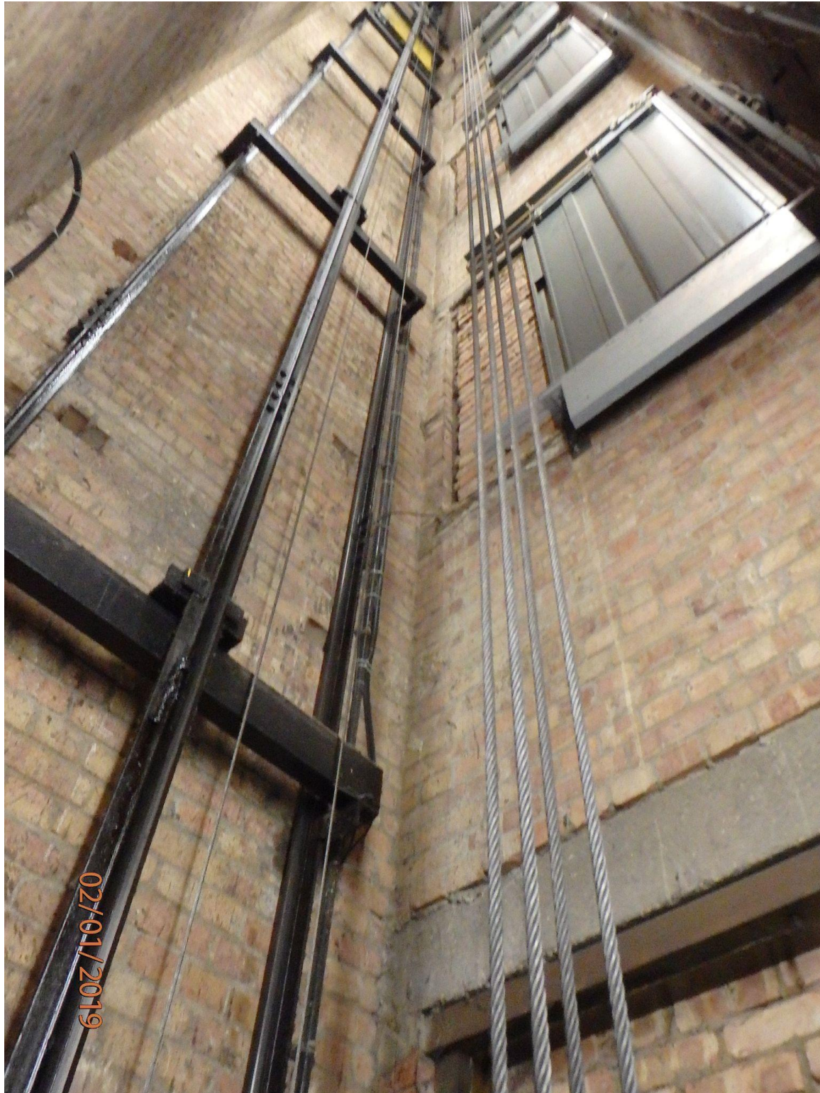
Interior (Lift Shaft) Existing lift shaft to building, currently serving Basement
