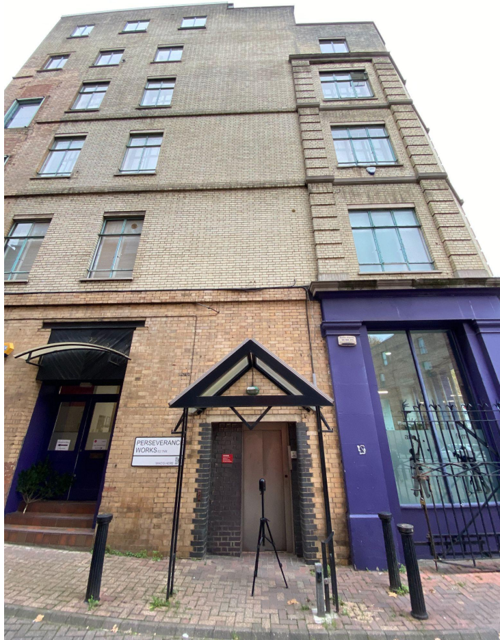
Exterior Secondary side access and external lift entrance
