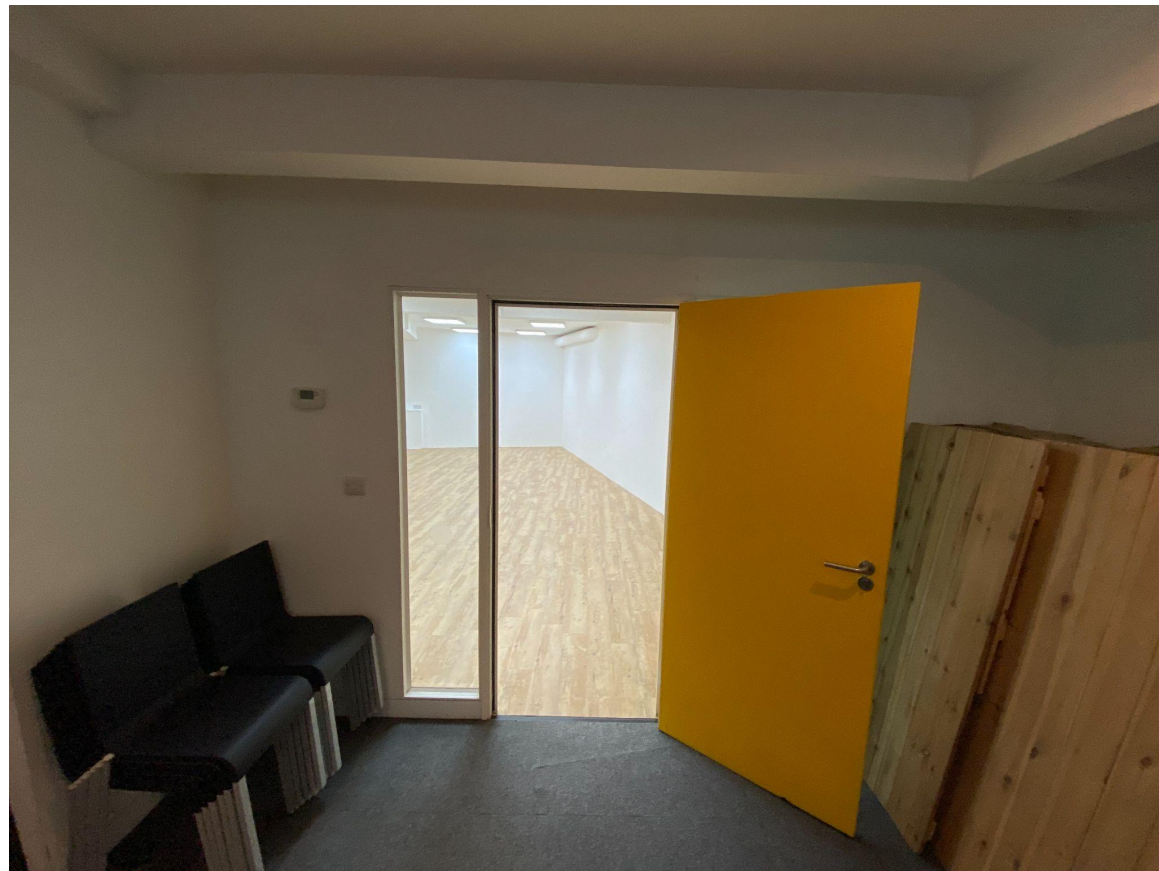
Interior (Basement) Door to main studio space from meeting space
